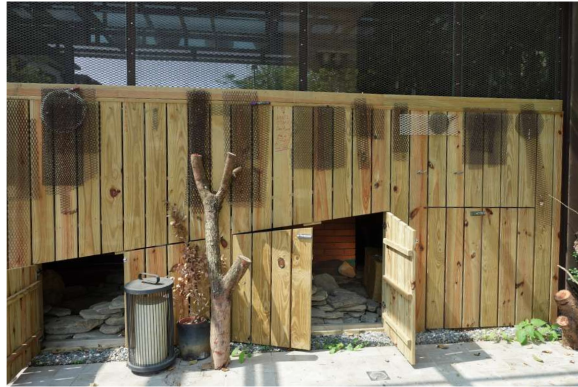
Fig. 1: The fence was cut along the level of the ramp, with the bottom part cleverly made into several disguised doors, which allow access to the space under the ramp.
