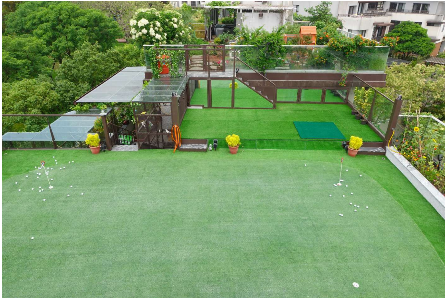
Fig. 7: From a bird's eye view, the structure linking the two roofs are clearly shown. At the top of the photograph is the wildlife garden rooftop, the bottom half is the newly built artificial putting green, and the section in-between is securely connected by a layer of bullet-proof glass, supported by solid metal pillars underneath.
