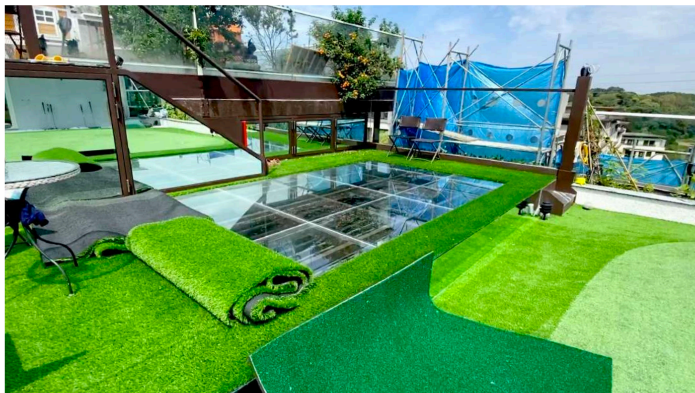
Fig. 2: On the side deck, artificial turf with longer grass was chosen, for one to provide a more realistic floor for chipping practice, and for another to create a relaxed atmosphere during social or family gatherings.
