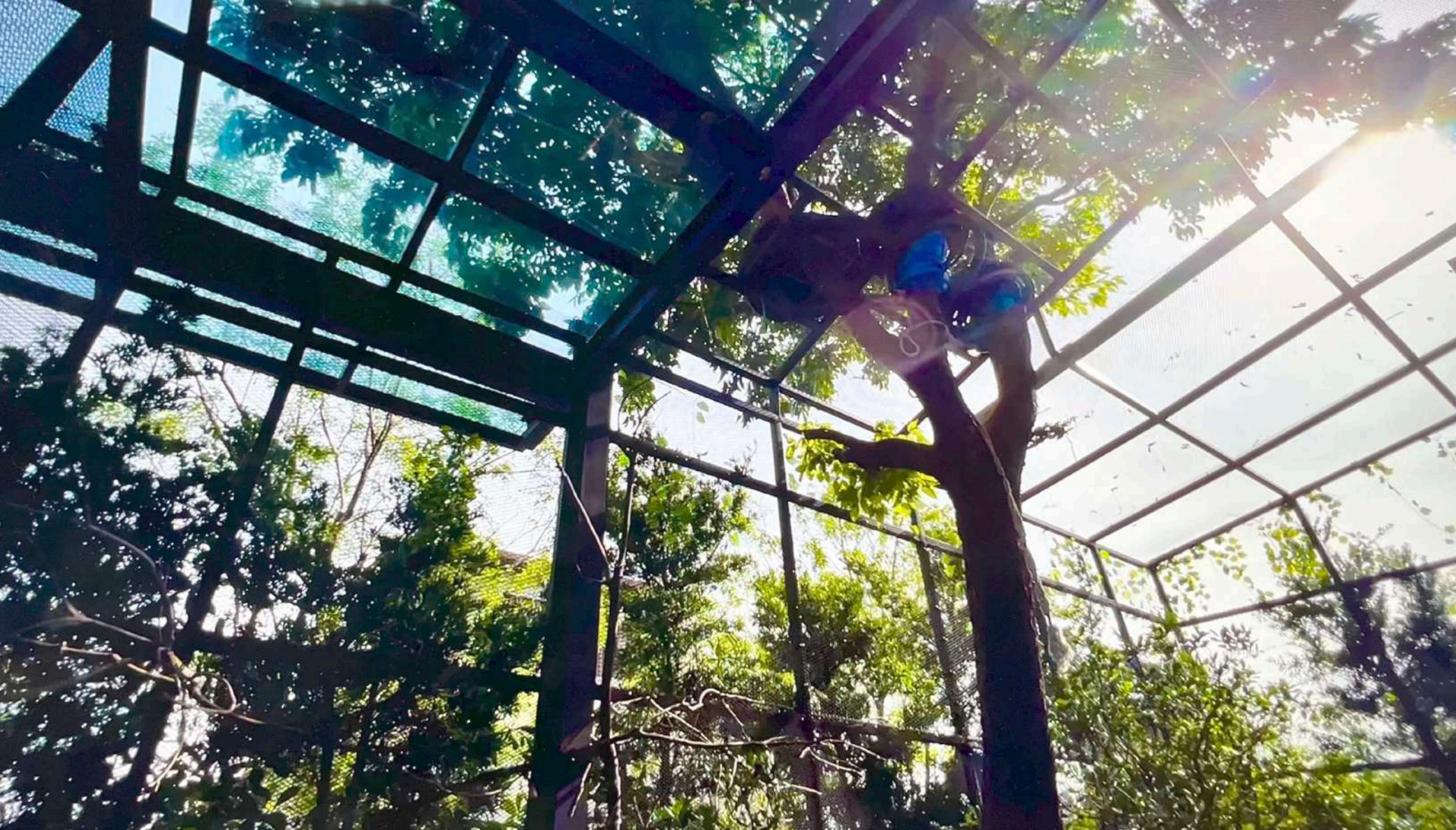
Fig. 1: With a 20-year-old bishop wood, which extends beyond the mesh of the aviary, a hard+soft approach was taken during the closing of the ceiling around the tree trunks. The metal frames should reserve enough spaces around the trunks, with soft, flexible materials (such as wasted tires, canvases, hoses, ropes, etc.) neutralizing the compression formed at the connecting points.
