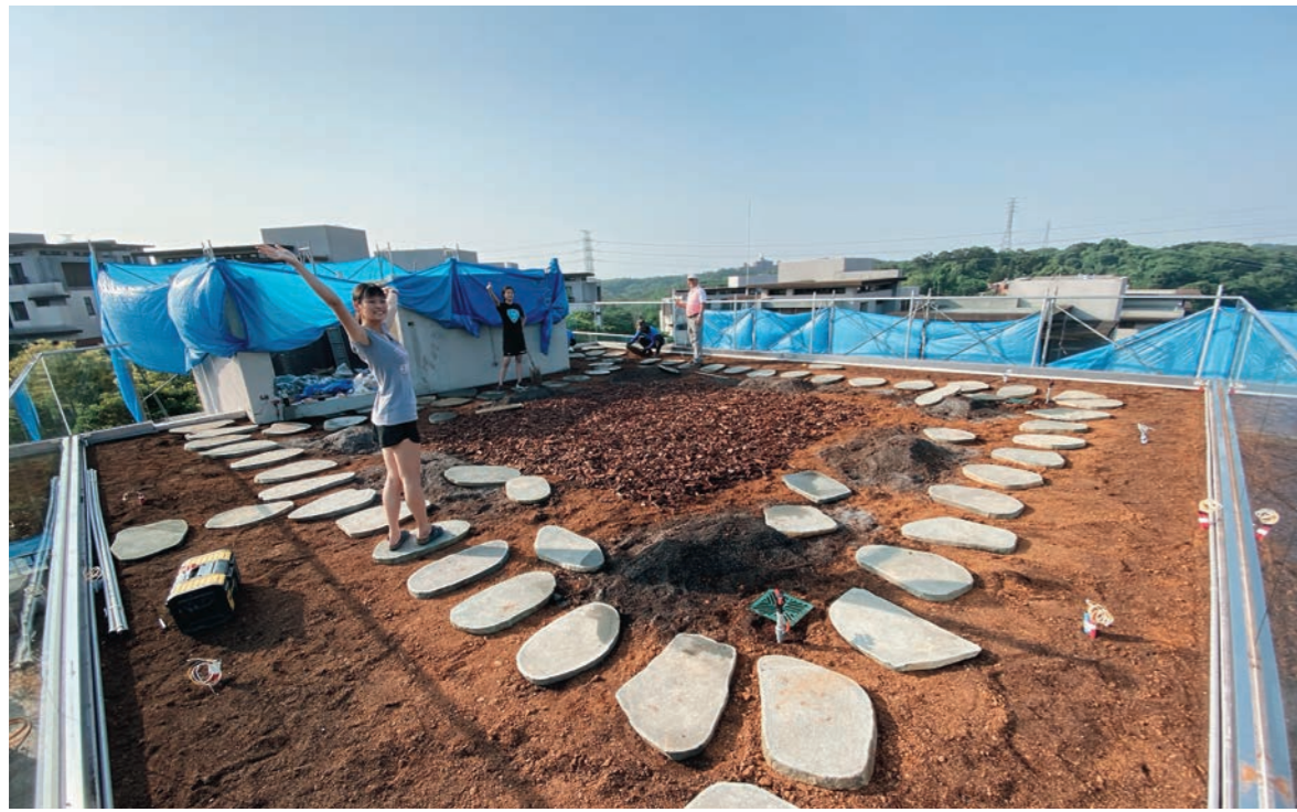
Fig. 6: The weight of the different materials making up planting medium has to be taken into consideration during distribution: heavy materials around the edges, and light ones in the center. Stone panels are arranged onto the soil as a walkway after planting is completed.
