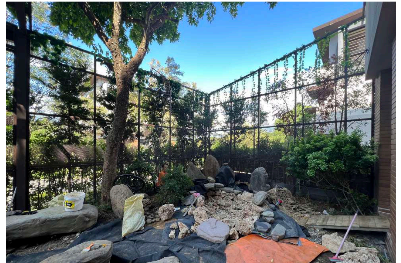
Fig. 5: For practicality, different liners were used to build the pond; however, they are nowhere to be seen in the completed landscaping. The devil is in the details, just like how the finishing steps in orthodontic treatment are what elevate the outcome from good to great.
