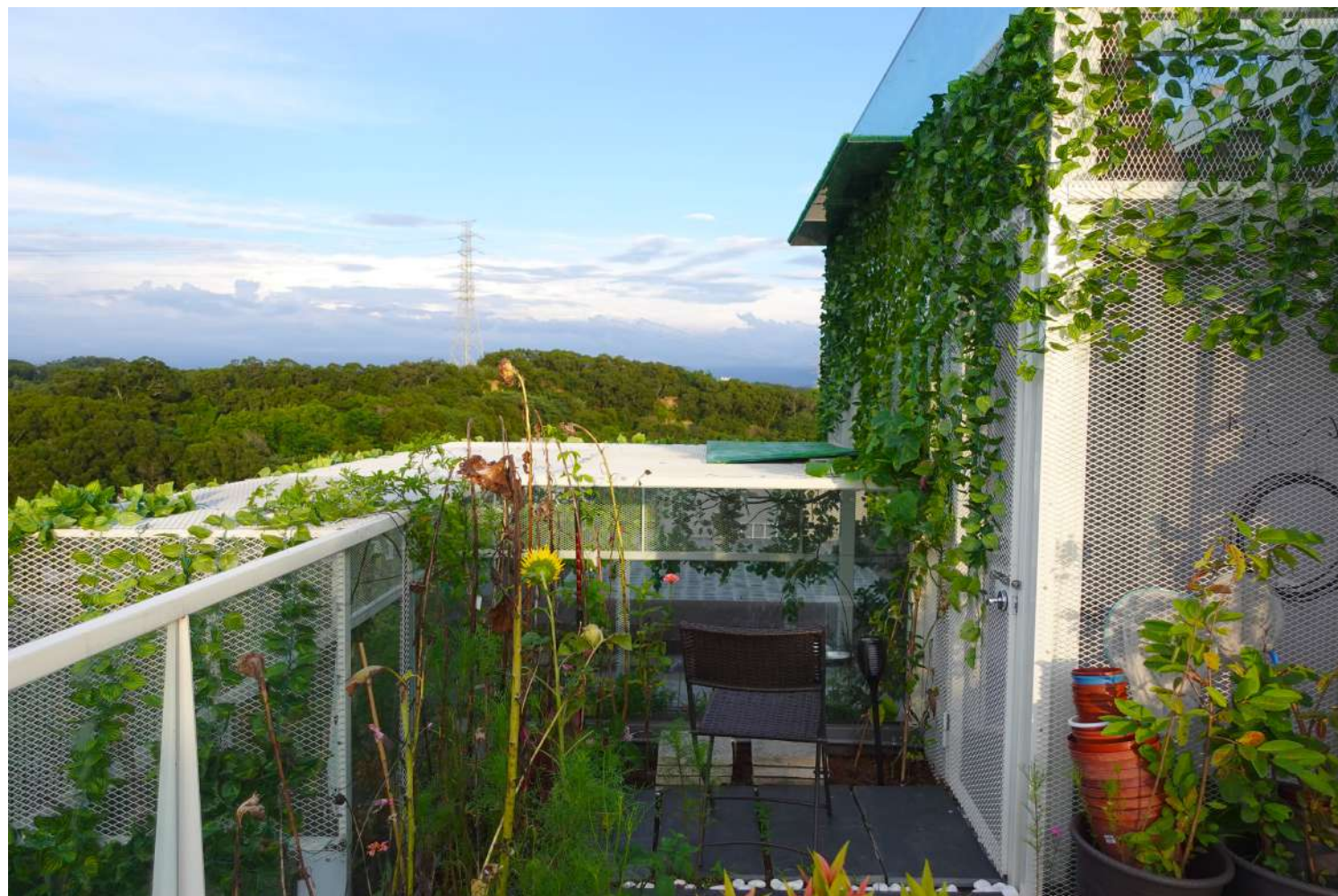
Fig. 1: Mesh walls and ceiling allow extended application of the vertical space in the aviary. In a practical sense, ventilation and shading can be created naturally. Attachment of auxiliary perches and climber plants is also made relatively easy, which enhances not only the functionality, but the playfulness and esthetics of the aviary.
